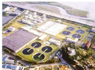
| Ilsan sewage treatment plant (135,000 tons per day)
