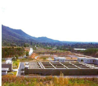
| Chiang Mai water supply facilities, Thailand
