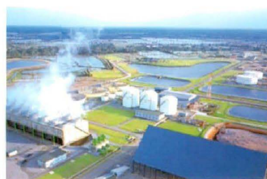
| Ratchaburi water treatment facilities, Thailand
