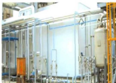
| Pipng work around A.W.U
