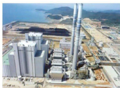
| Yeongheung thermal power plant #1,2 electrostatic precipitators (800MW x 2)
