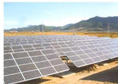
| Solar Energy Power Plant Construction (5080MWH)
