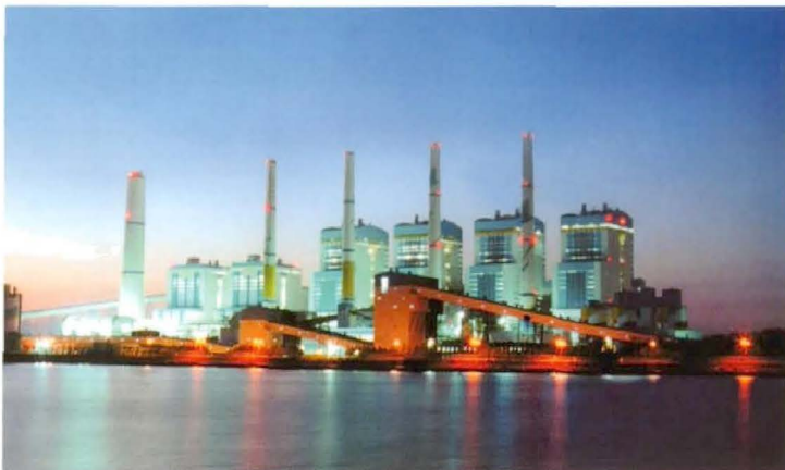
Taeon Thermal Power Plant (7, 8 units)
