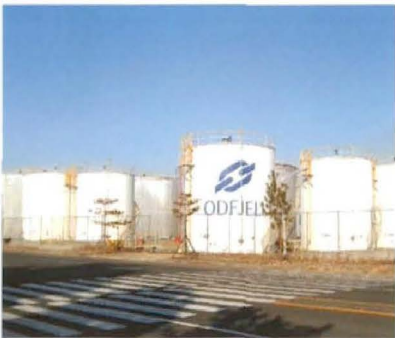
ODFJELL Terminal in Korea installed all WBIFR on tank farms
