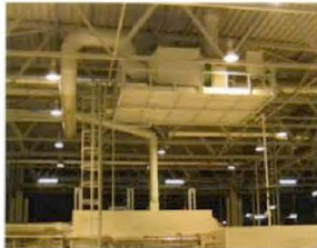
Automobile Engine Factory of the Europe Office - Oil and water soluble OIL MIST dust collector
