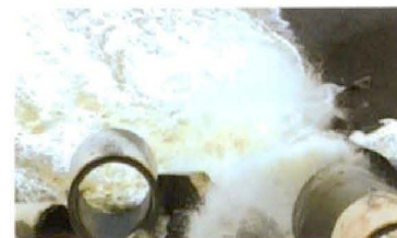
| Pre-treatment of the desalination of seawater
