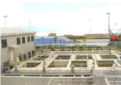
PACIFIC GLASS (AMORE) - Wastewater treatment construction
