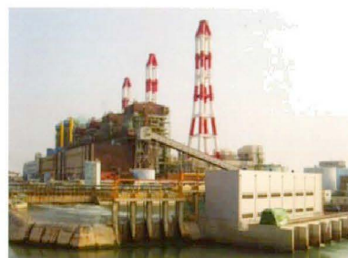
| Samchenpo small hydropower generation facility(1,000 KW x 6)
