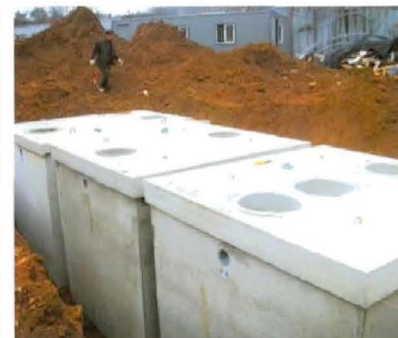
| After the attachment of the upper plate
