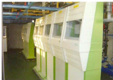
Sewage processing facility
