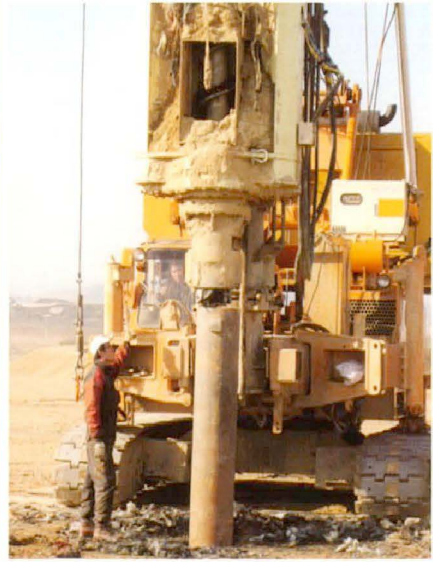
Boring vertical infiltration well by Auger
