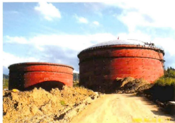
Aluminum Dome Roof for Oil Storage Tank, Algeria (Dia52m x 2Sets)
