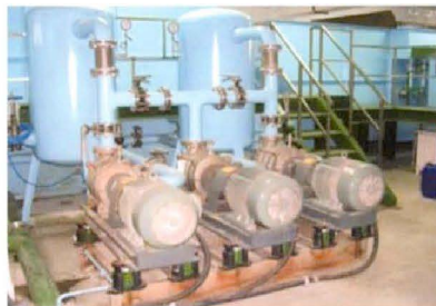
Banwol Plating Industry Cooperative - Wastewater treatment construction
