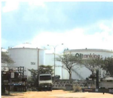
Oiltanking Terminal, Singapore (Aluminum Dome, Seal and Drain systems)
