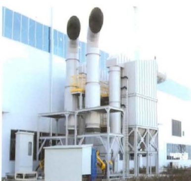
2000CMM Dust Collector (Long-round type cartridge filter)
