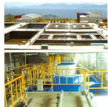
Biological treatment facility
