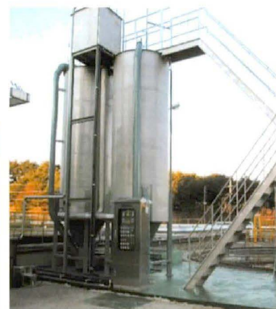
PASTEUR - Wastewater treatment construction
