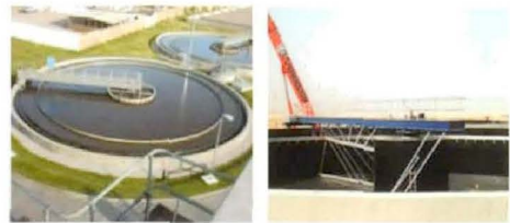
| Circular sludge collector
