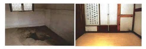
An ondol, also called gudeul, in Korean traditional architecture, is underfloor heating system which uses direct heat transfer from wood smoke to the underside of a thick masonry floor.
