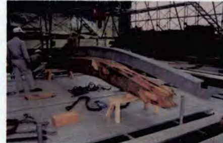
Steel beam added in the Wooden beam
