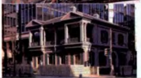
△旧居留地十五番館(災害復旧) After Restoration
