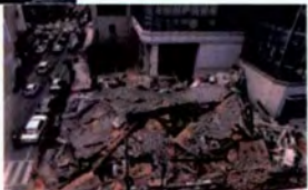
△旧居留地十五番館(被災状況) Before Restoration
