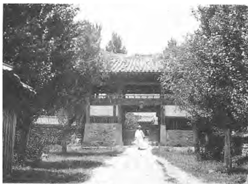
Facade of Ich'on Police Station.
